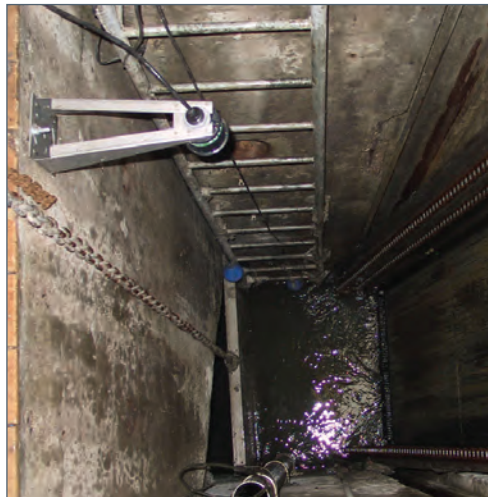
WET WELL 6m WITH LADDER AND FLOAT
