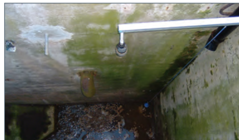
HINGED BRACKET OVER A WET WELL
