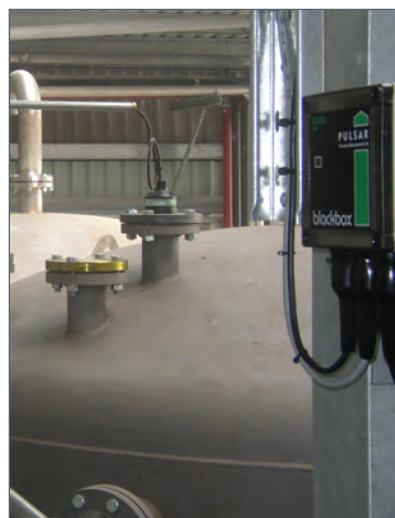
FLANGED TRANSDUCERS SHOWN ON TANKS
