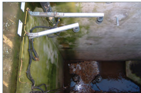
HINGED BRACKET OVER A WET WELL
