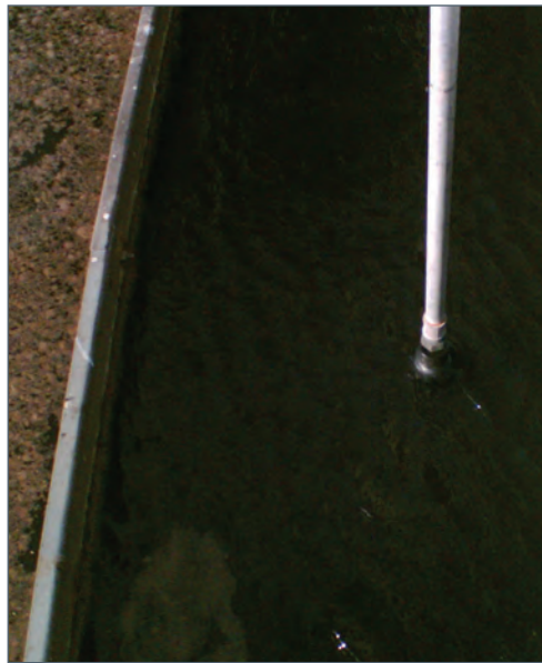
VIPER MOUNTED BEHIND SURFACE SKIMMER AND IN FRONT OF ROTATING BRIDGE
